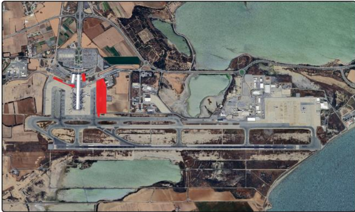
Figure 1-3: Satellite view of Larnaca Airport Extension Project (Source: BBI-Egis Avia, December 2023)
